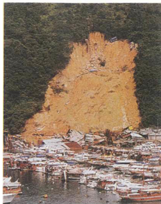
Shum Wan Road landslide
