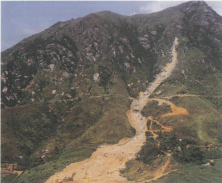
Fig. 5.5 An unstable slope in Castle Peak
