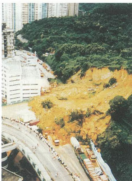
Fig. 5.11 A road blocked by a landslide
