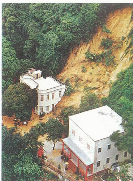
Fig. 5.10 A temple in Sha Tin damaged by a landslide
